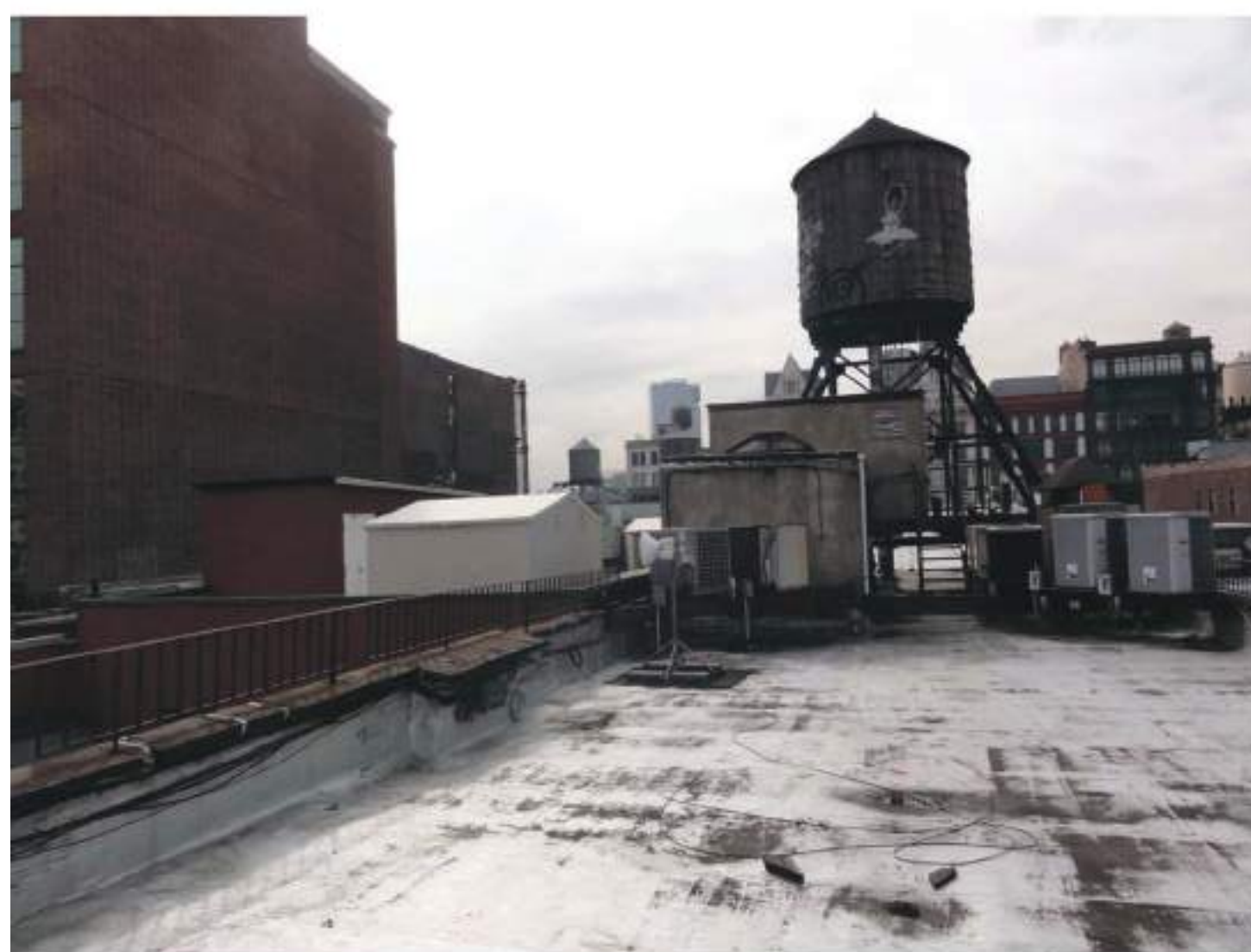
4 EXISTING ROOF (EAST VIEW)
