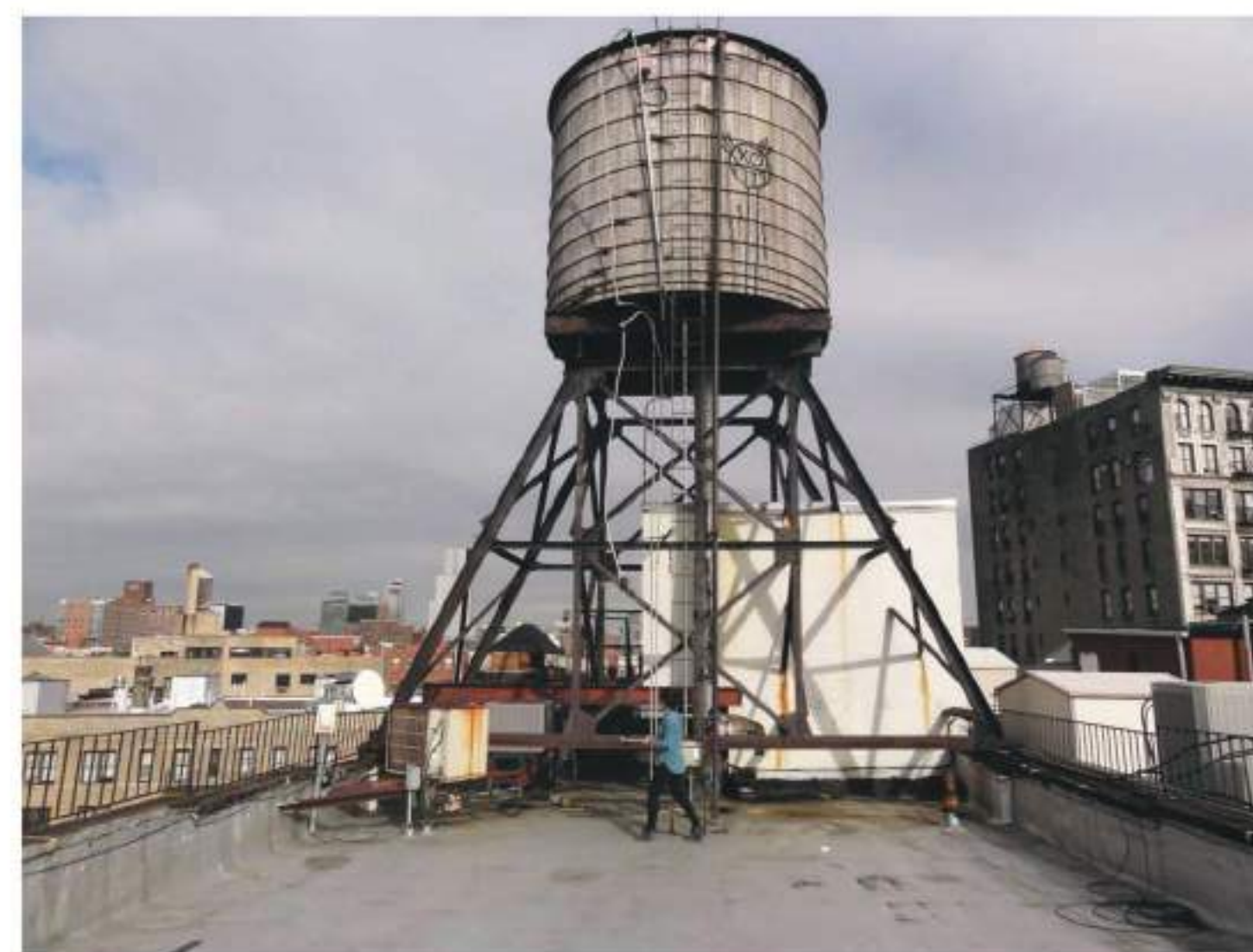
5 EXISTING ROOF (WEST VIEW)
